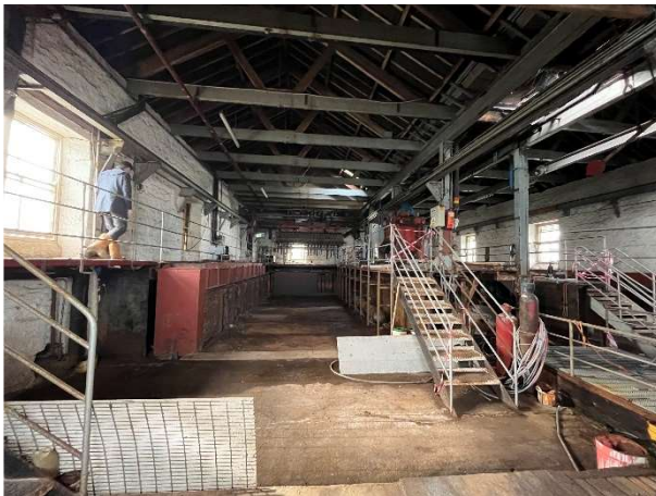
Second floor level showing roof structure
