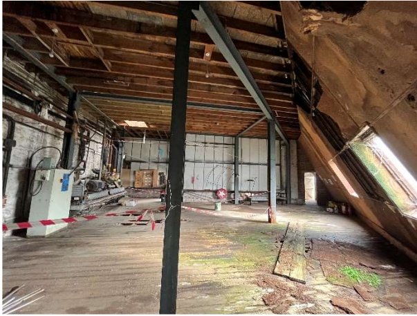
First floor level showing roof structure
